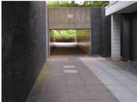
Photo 18: Underpass below Northway
