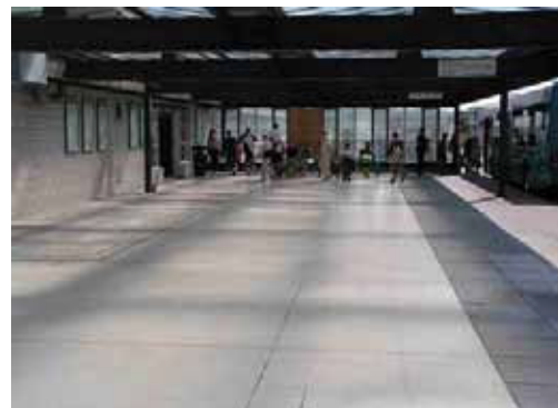
Photo 8: Northern Bus Terminus
