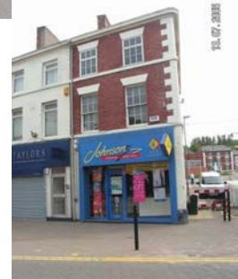
Church Street South side unit with non- standard Frontage treatment
