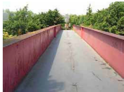
Photo 2: Footbridge towards Asda
