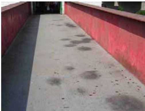
Photo 20: Surface of footbridge from East Lane House.
