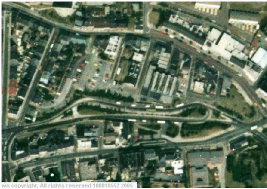
Aerial view of Central Area in 1983 showing the elaborate busway interchange severing linkages between Church Street (top) and High Street (bottom).
