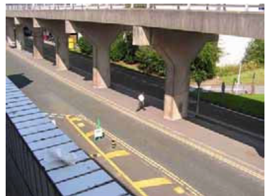
Photo 3: Pedestrian crossing road at ground level
