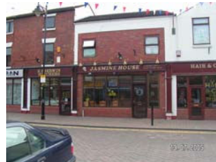
Church Street : Southern units showing uniform frontage treatment
